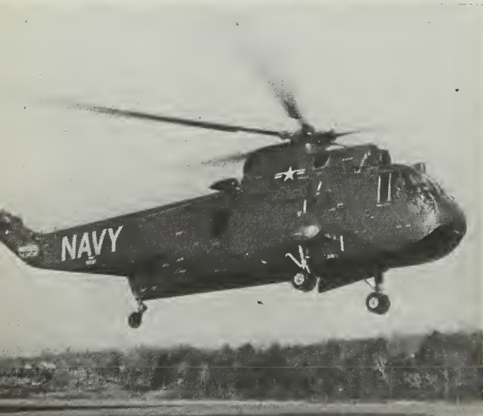
WATER BIRD —New gas-turbine-powered copter with choice of boat hull or wheels can land almost anywhere.
